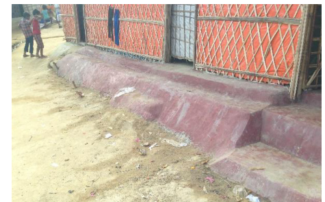
Plinths in Cox's Bazar. IOM (2018b) Catalogue of site improvement
