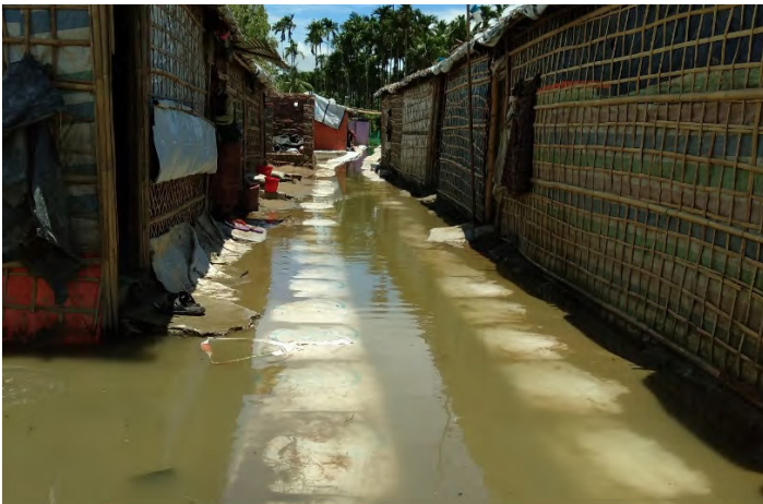
Trapped water when drainage outlet was blocked near Cox's Bazar (IOM, 2018c)
