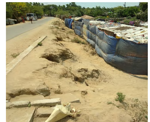
Embankment erosion (IOM, 2018c)
