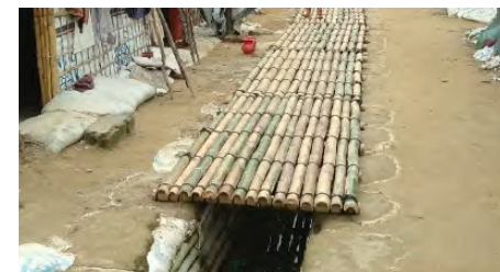
Covered channel in Cox's Bazar (IOM, 2018c).
