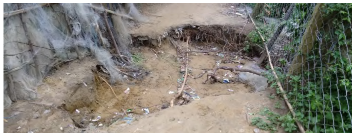
Road damaged by water runoff at high level areas near Cox's Bazar (IOM, 2018c)
