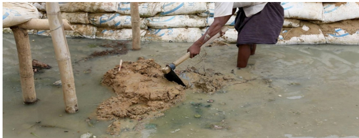
Clearing silt-clogged drainage canals to stop flooding and contamination of clean water sources in Cox's Bazar (IOM, 2018c)
