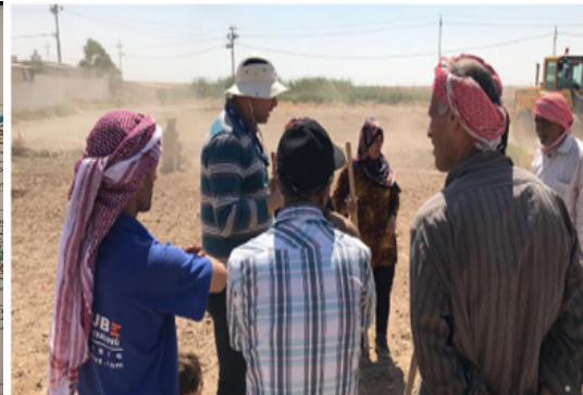
A site walkover with UNHCR WASH Associate, camp management and women from the SuDS community committee was conducted.
